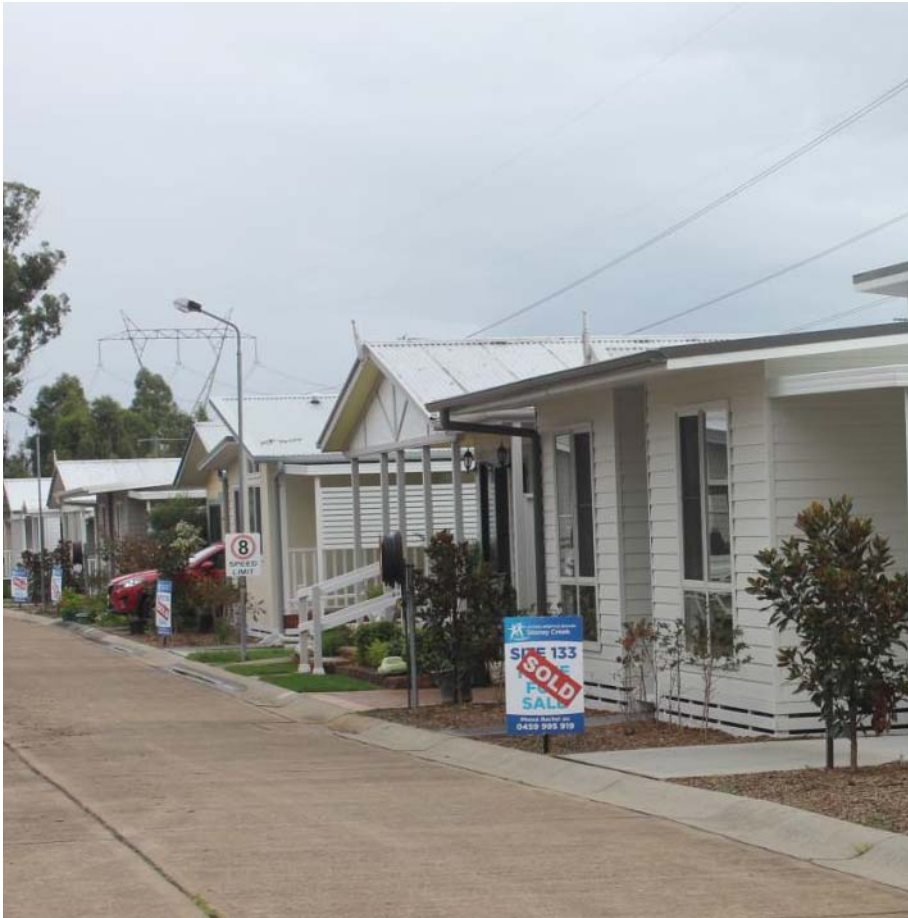
Stoney Creek Estate, Marsden Park (Sydney)
