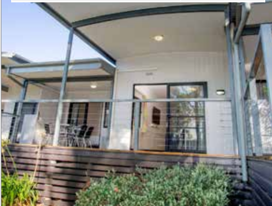
Ingenia South West Rocks, NSW
