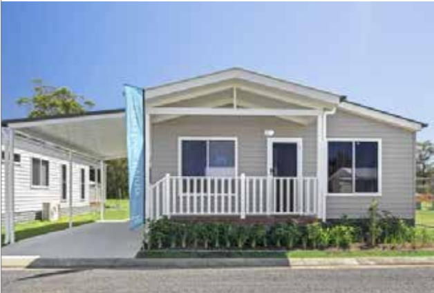
Ingenia South West Rocks, NSW
