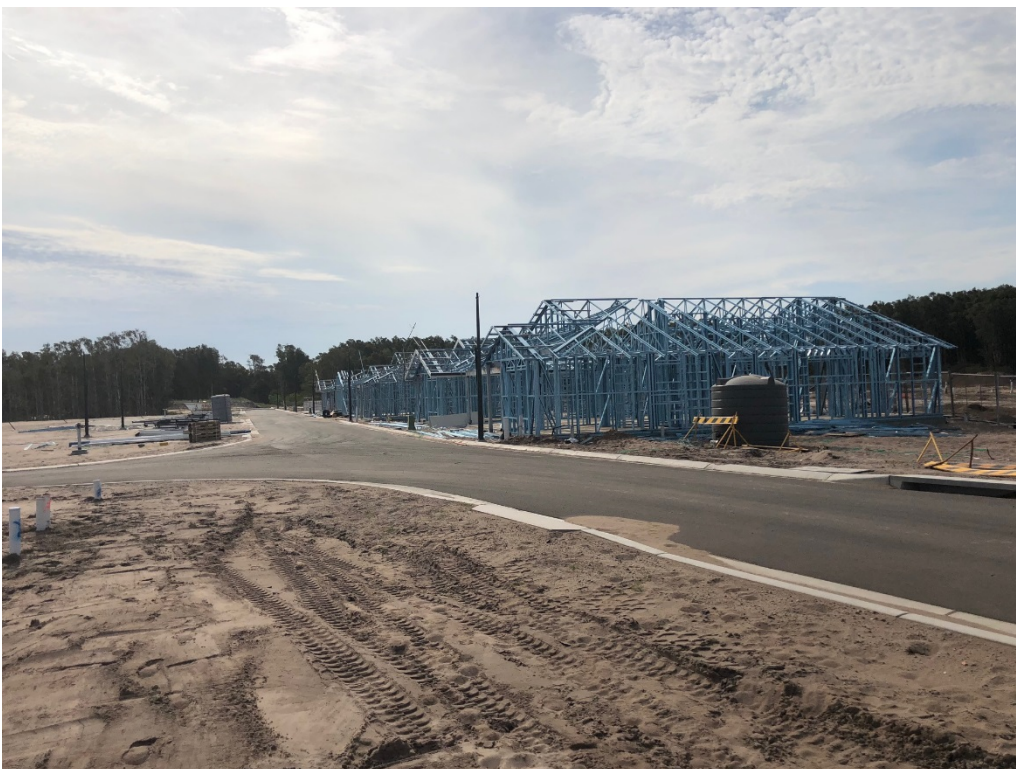
New homes under construction at Latitude One.
